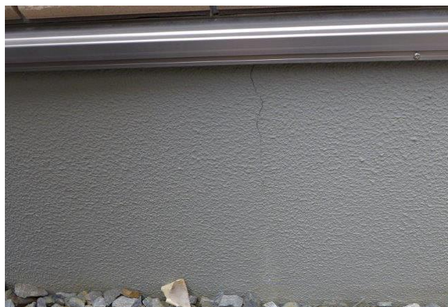
ひび割れ幅は0.4mm
